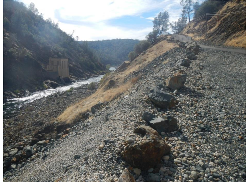
Figure 5: Photo of Narrows 2 access road and erosion scars looking downstream (Oct. 30, 2014).
