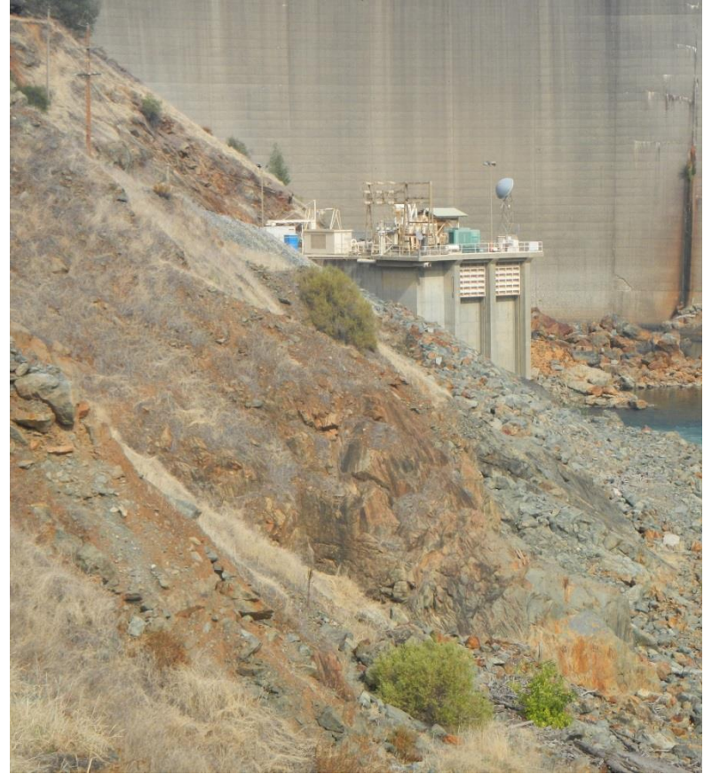
Figure 7: Photo of Narrows 2 and shot rock supporting Narrows 2 access road (Oct. 30, 2014).
